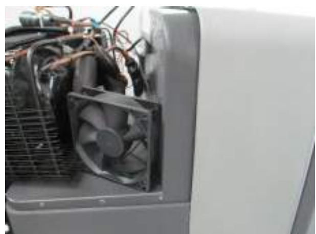
6. Remove the fan and reverse the procedure to install the new fan
